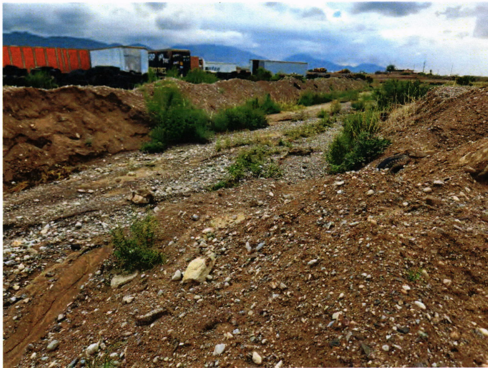
Photograph 12 – 1-4 MID moist, no standing water, within an active construction site (8/18/2022).
