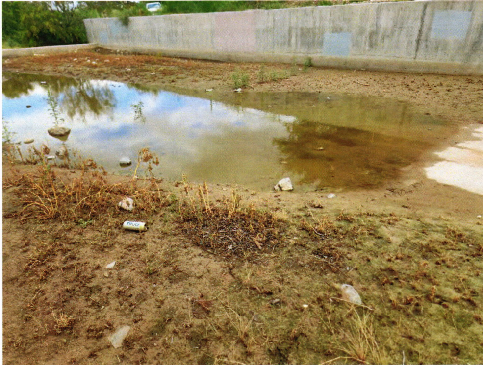
Photograph 13 – 1-5 MID, standing water (8/18/2022).
